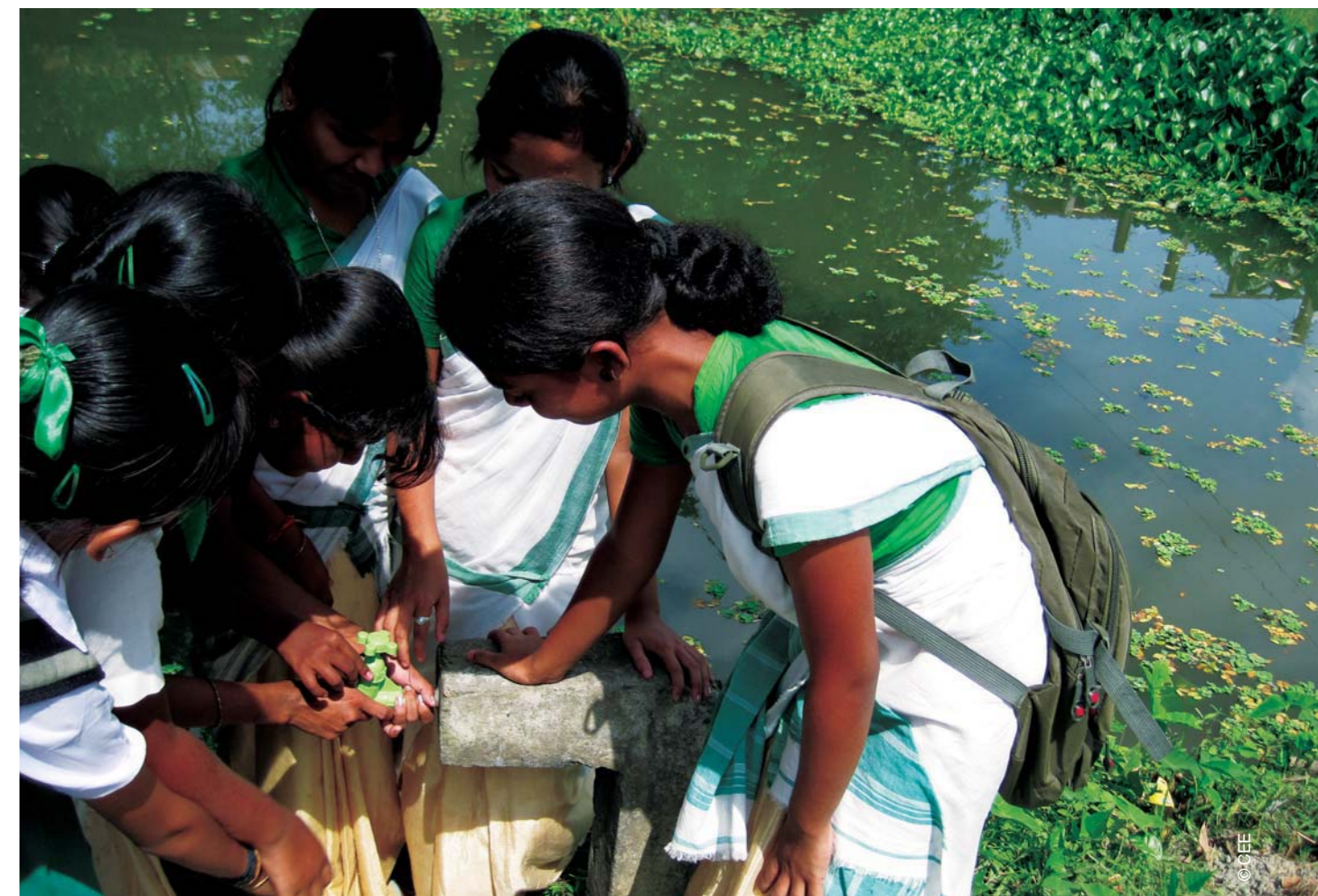
△ Students fitting water tap to a stand post (North Ghy)
