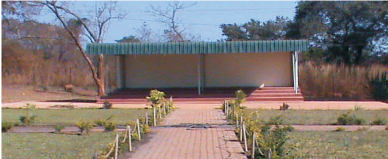
Figure 5: Graduation Podium Constructed with help of students.
